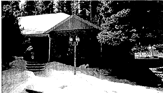
2-21-11, FRONT VIEW (NW)
