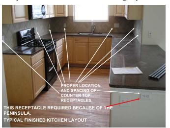
On or above the countertop or work surface: On or above but not more than 20" above the countertop or work surface. [210.52(C)(3)(1)] In countertop or work surface: Receptacle assemblies, must be listed for the purpose. [210.52(C)(3)(2)] Below countertop or work surface: Cannot be more than 12" below the countertop or work surface. Receptacles shall not be installed where the countertop or work surface extends more than 6" beyond its support base. [210.52(C)(3)(3)]
