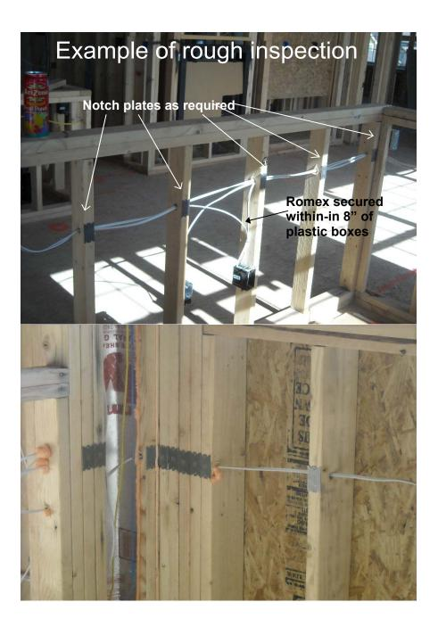
NM (romex)cable must be installed 1-1/4" back from the nearest edge of the hole in wood members or protected by 1/16" steel sleeve or plate. [300.4(A)(1)]
