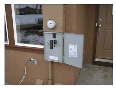
The electrical installation shall be complete at the time of request. The "temporary building service"/permanent power meter is set, service equipment complete and labeled properly. All wiring shall be free from short circuits, ground faults, and open circuits. All light fixtures are required to be complete (i.e. Lensed, glass, trims, and lamps installed) and grounded along with light switches that are within five feet of a grounded object. All 120volt circuits shall have power.
