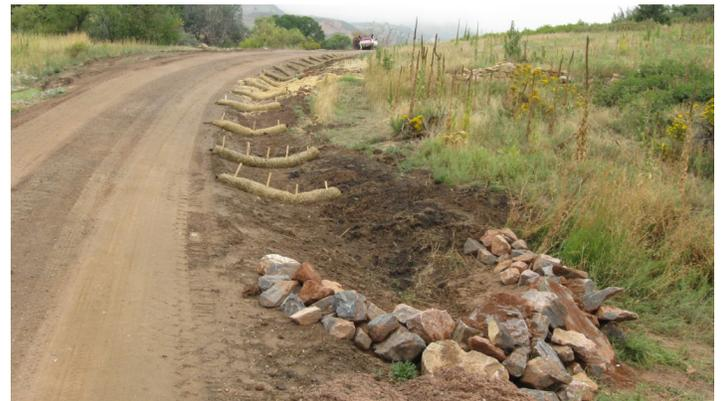
**Note:** Performance of sediment controls is dependent on proper installation, routine inspections and maintenance of the controls. Most of the BMPs described above are temporary and if left alone, can quickly fall into disrepair and/or become ineffective. Routine inspections and maintenance, particularly before and after a storm event, must be part of an erosion and sediment control plan.
